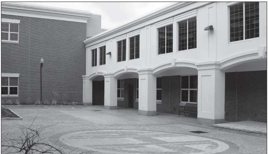
New central courtyard surrounded by both the new addition and the old building
