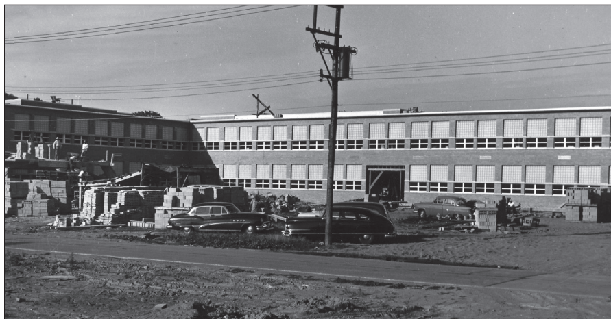
Henderson east side construction 1954
